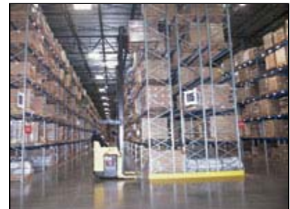
Warehouse space at TIC features an ESFR-plus sprinkler system and clear heights between 50 and 70 feet.
