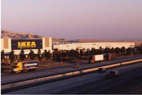
IKEA Distribution Center
